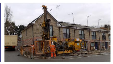
This was an Emergency Investigation and Treatment Works Contract which was undertaken following the formation of a ground collapse directly outside a property on this newly constructed housing development in Plumstead, South East London. The residents adjacent to the collapse were immediately evacuated and the initial collapse filled with concrete. Peter Brett Associates were appointed by the client to design and supervise a site investigation followed by a ground treatment scheme.
